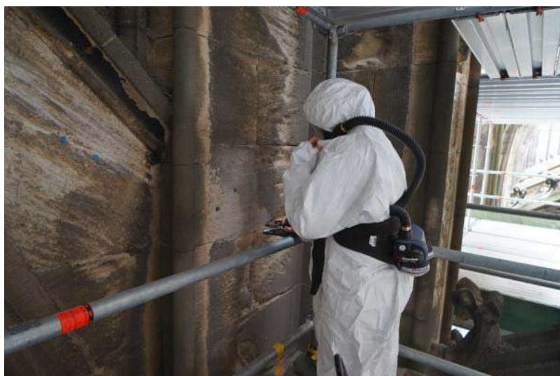
Illustration 28: Sandblasting at the façade of Cologne Cathedral, Source: Dombauhütte Köln, Foto: M. Wurth
