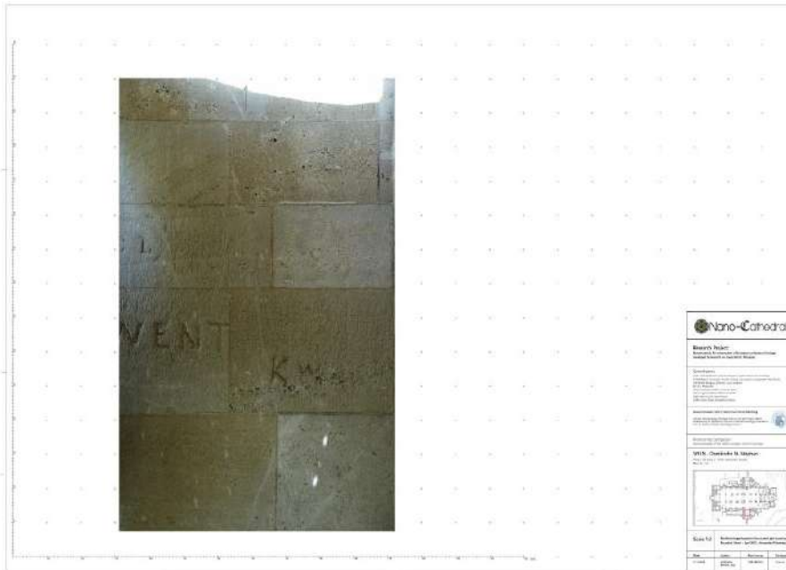
Fig. 09: General view of Trial Area 3_12 S.
