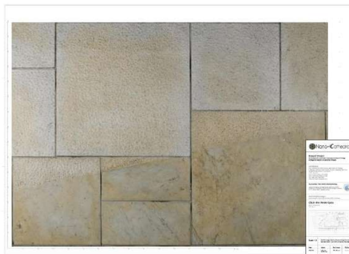
Fig. 02: General view of Trial Area P3A.
