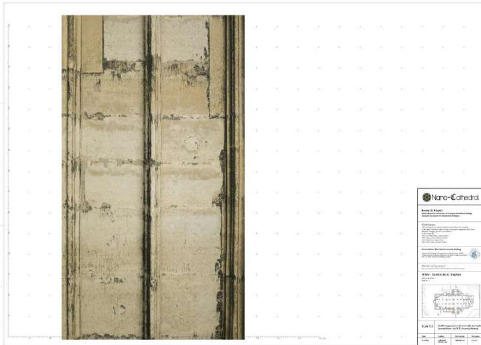
Fig. 01: General view of Trial Area 1 Part 1.
