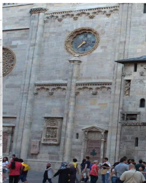
Oldest parts: ground floor and its
