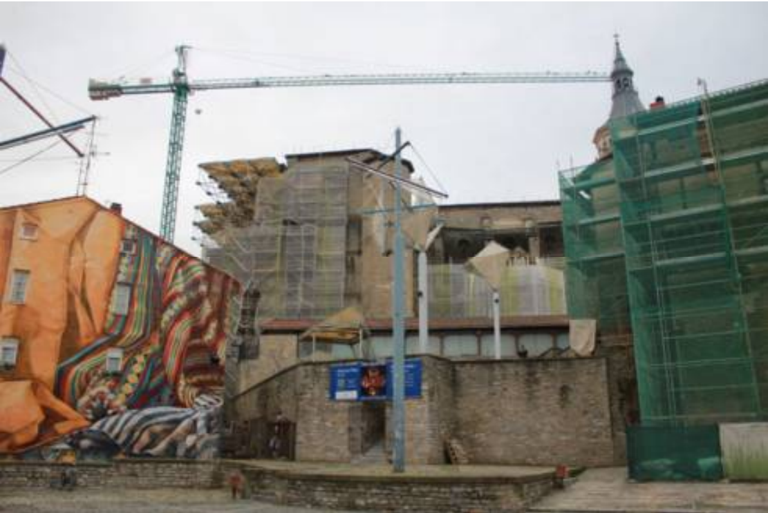
Northern facade of the transept
