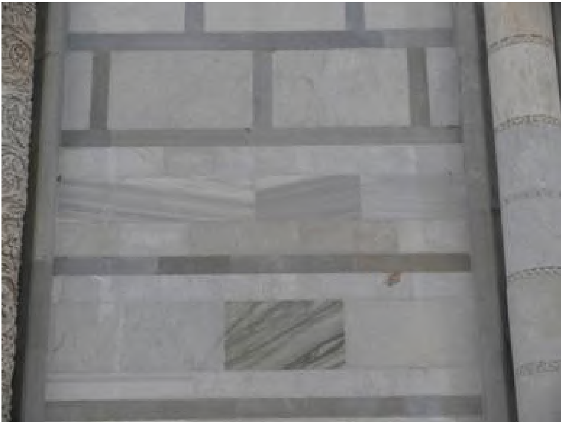
Detail of the façade wall
