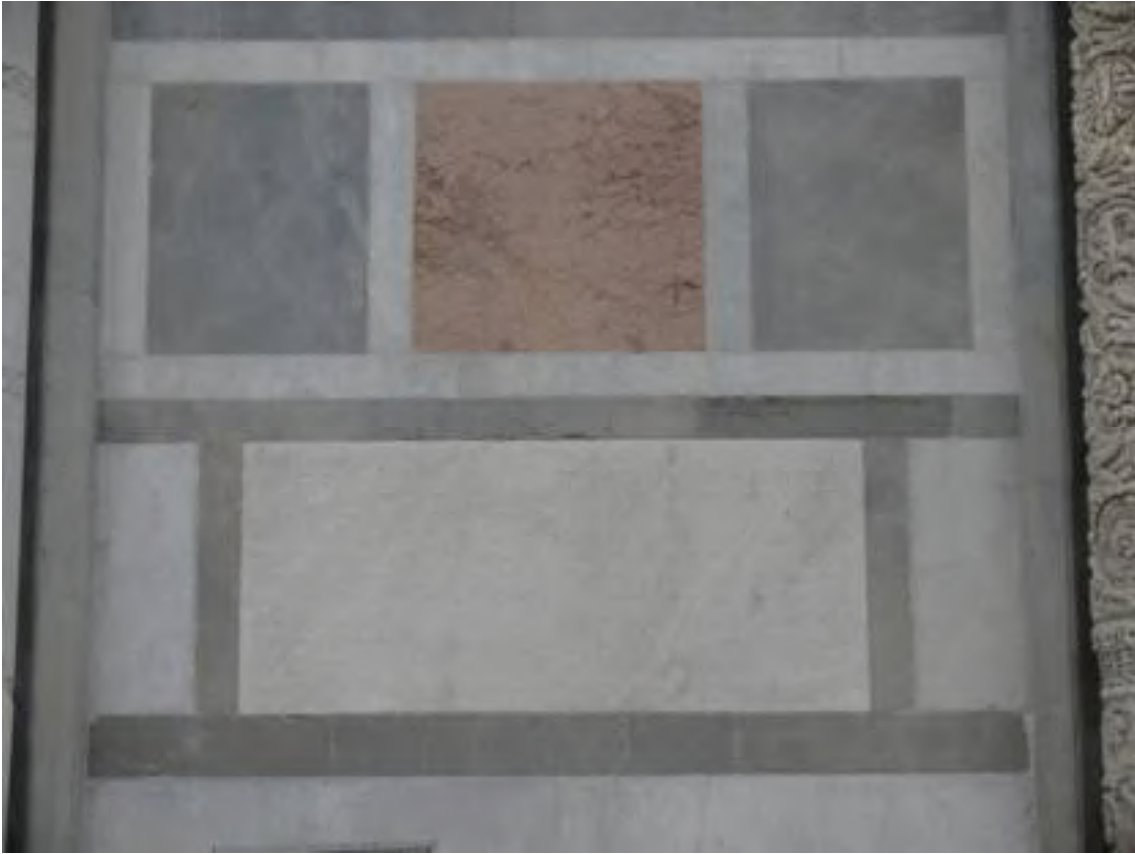
Detail of the façade
