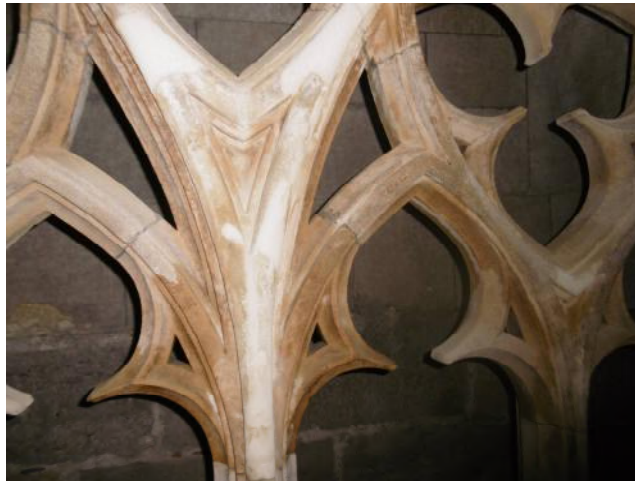
Tracery with linseed oil on the "Friedrichsgiebel"
