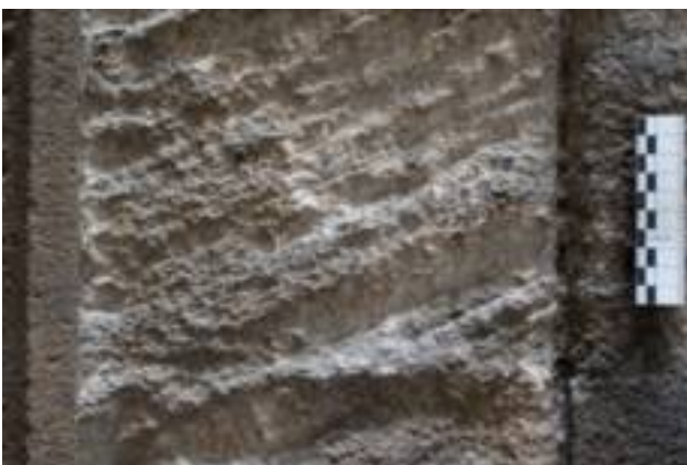
Fig. 13: Schlaitdorf Sandstone, detail, various specific damages like strongly sanding, delamination, crumbling, granular disintegration, black crusts.
