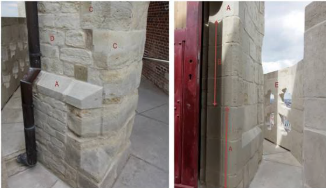
Image 26. Area's after restoration with (A) new pieces of Balegem stone, (B) cleaned and repointed Balegem stone, (C) new pieces of stone glued into the original Balegem stone, (D) cleaned and repointed Gobertange stone. The parapet is built in Massangis (E).
