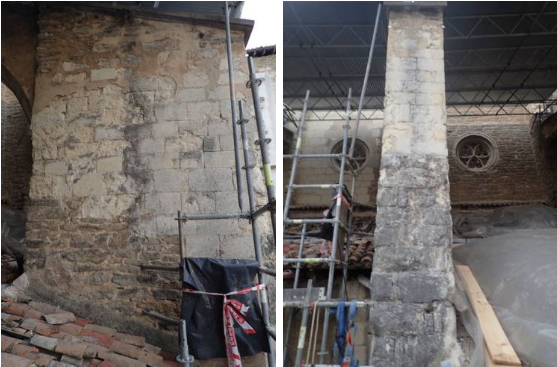
Buttresses of the transept
