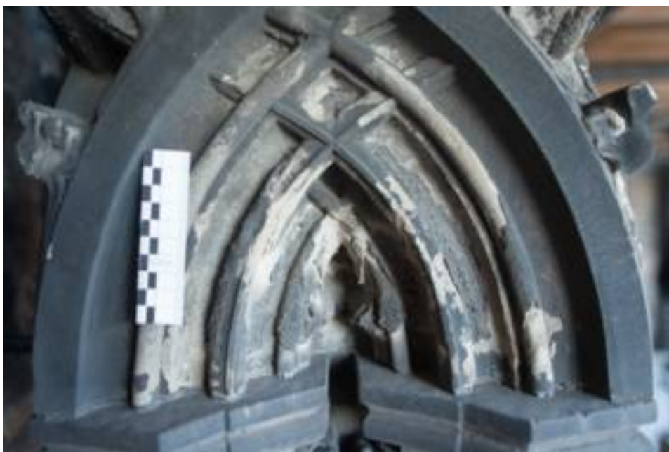
Fig. 15: Obernkirchen sandstone, detail, various specific damages like scaling, powdering, black crusts, exfoliation, flaking, soiling and powdering.
