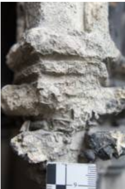
Fig. 11: Tercé limestone (details), various specific damages like microkarst, sanding, black crusts, exfoliation and soiling.
