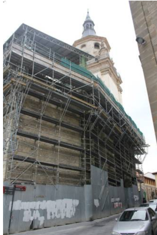
Exterior of the portico under scaffold
