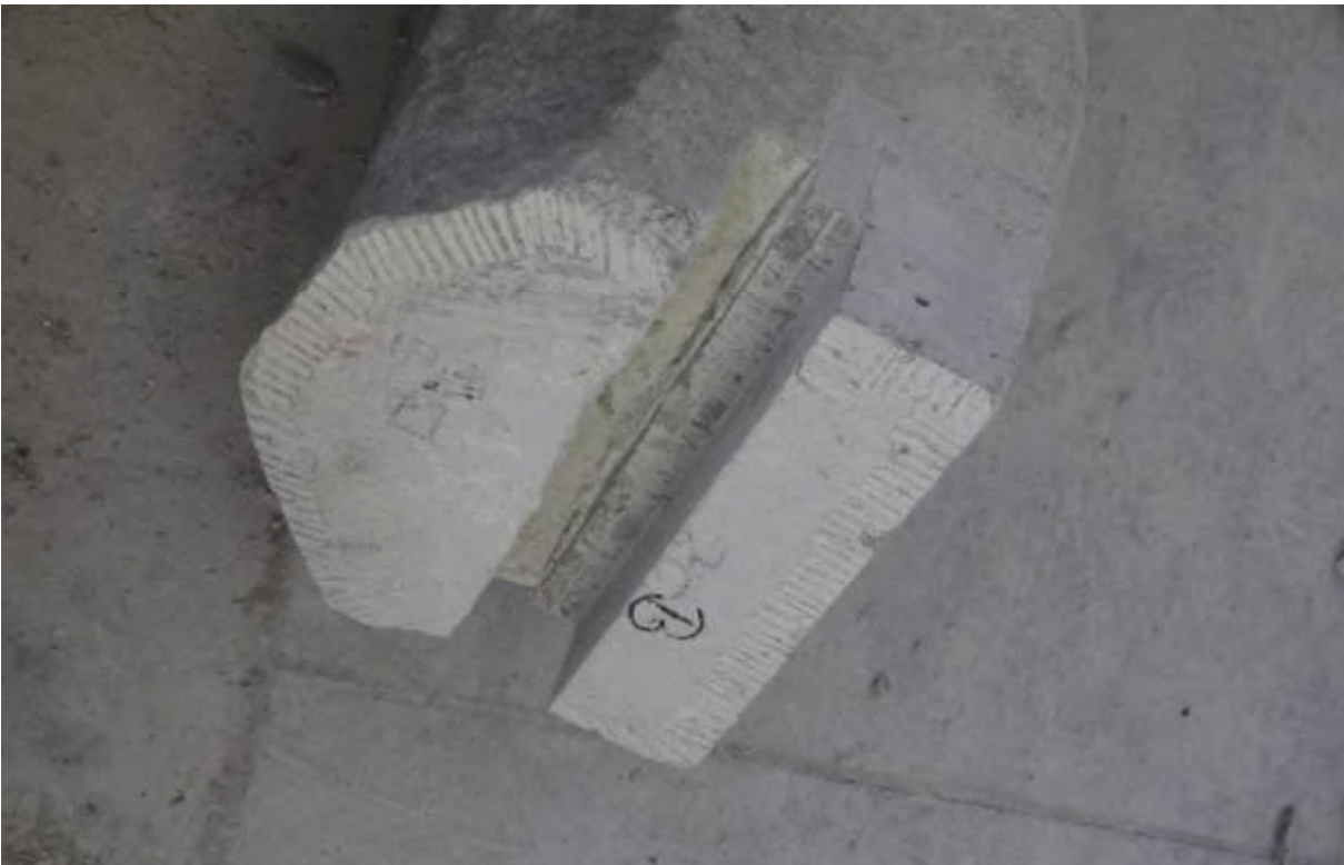
Image 23. New pieces of stone, glued into the original stone.
