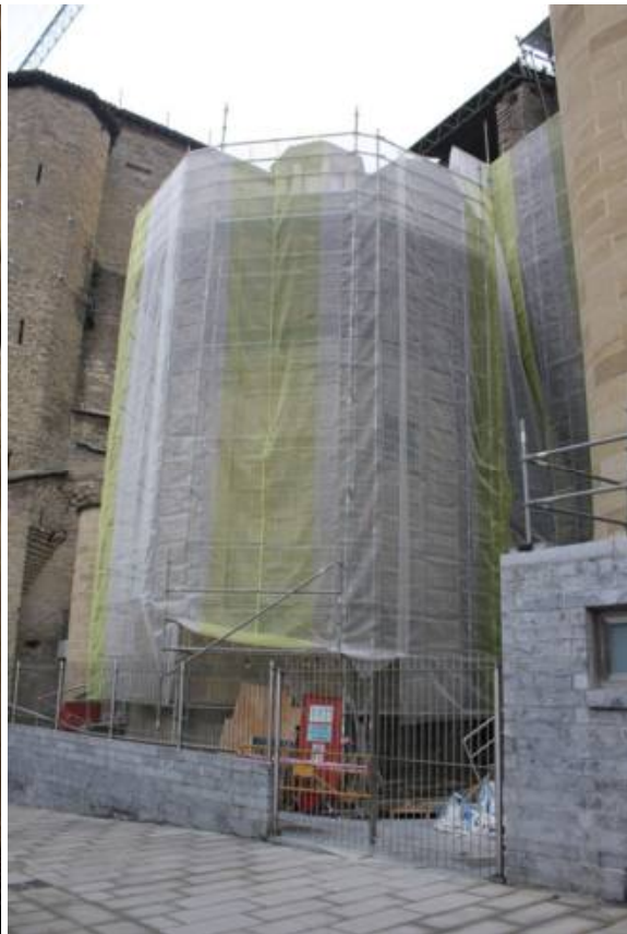
Northern facade of the nave under scaffold
