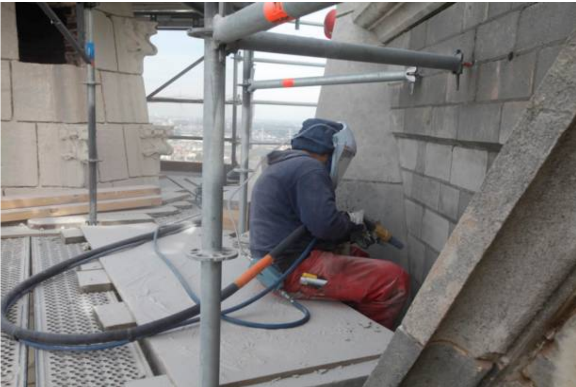
Image 24. Low pressure wet abrasive blasting with rotating nozzle.
