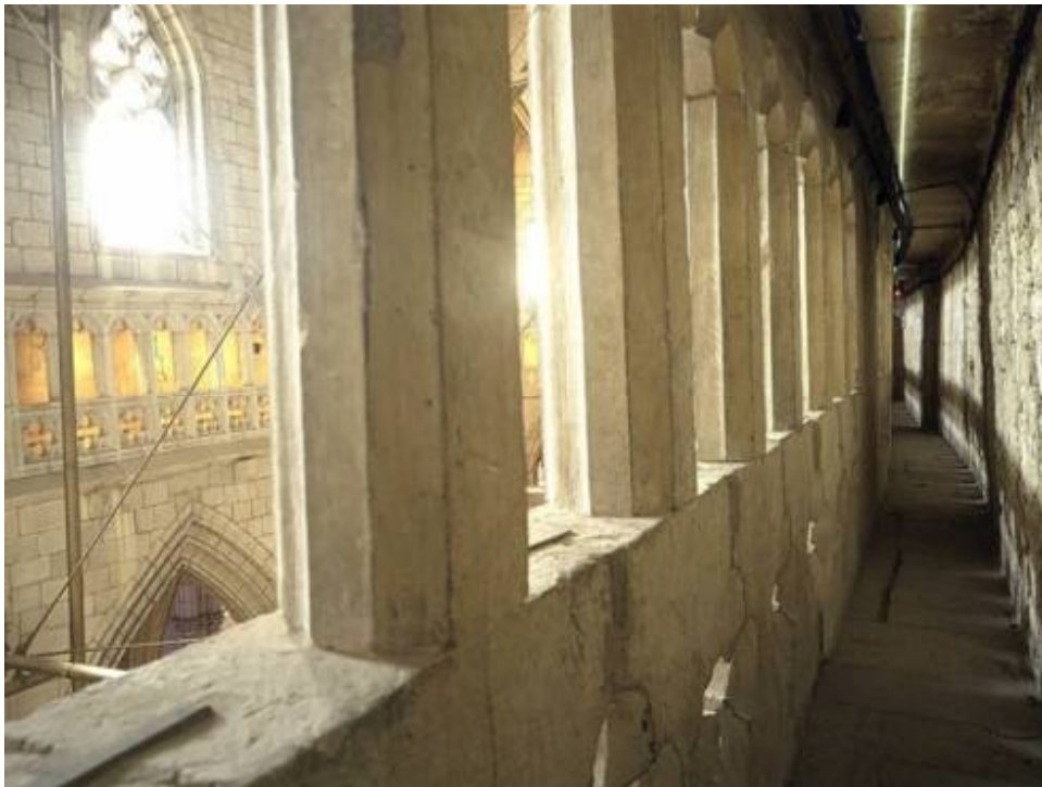
Interior gallery of the clerestory
