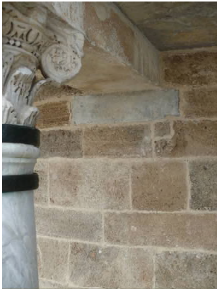
Third storey wall made up with Panchina calcarenite
