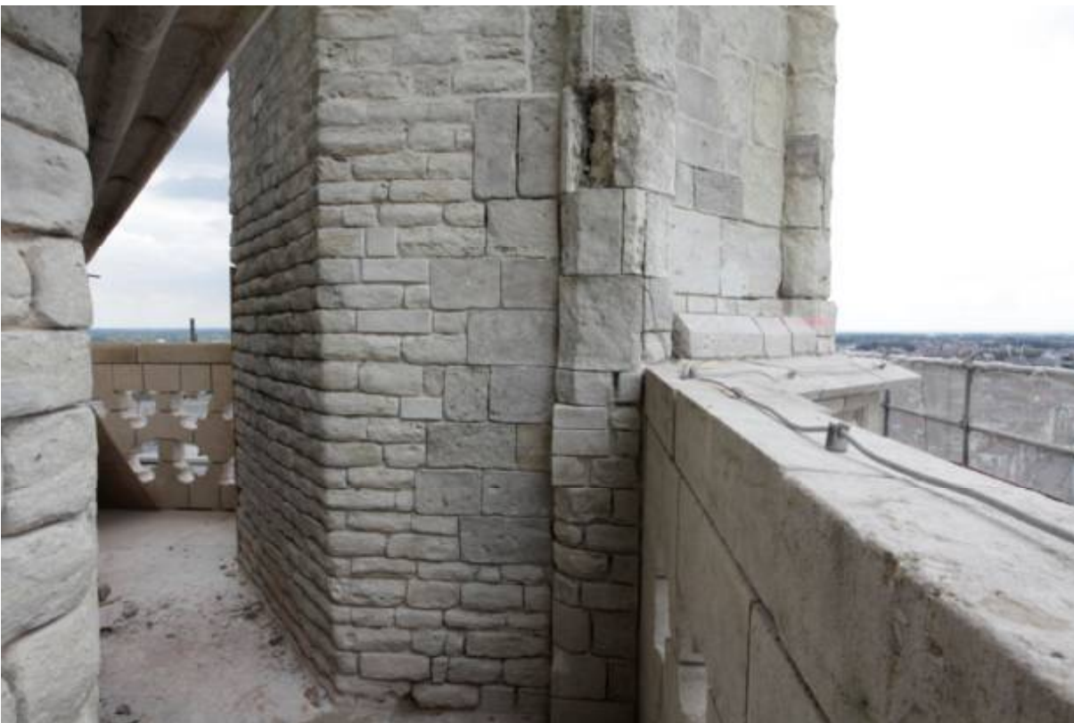
Image 25. Cleaned Gobertange (A) and Balegem (B) after the removal of the pointing.
