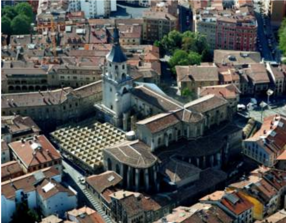
Catedral de Santa Maria: Aerial view from south east, with the transept and Santiago chapel
