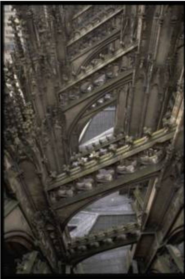
Fig. 6: Cologne Cathedral, buttressing of the south side.
