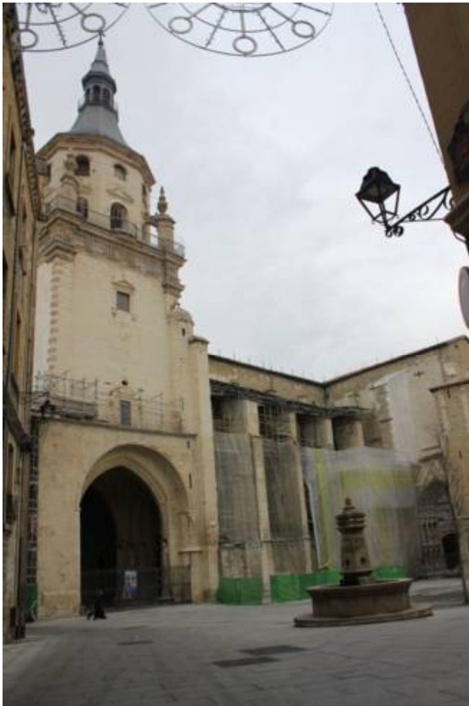
Southern facade of the nave with belfry
